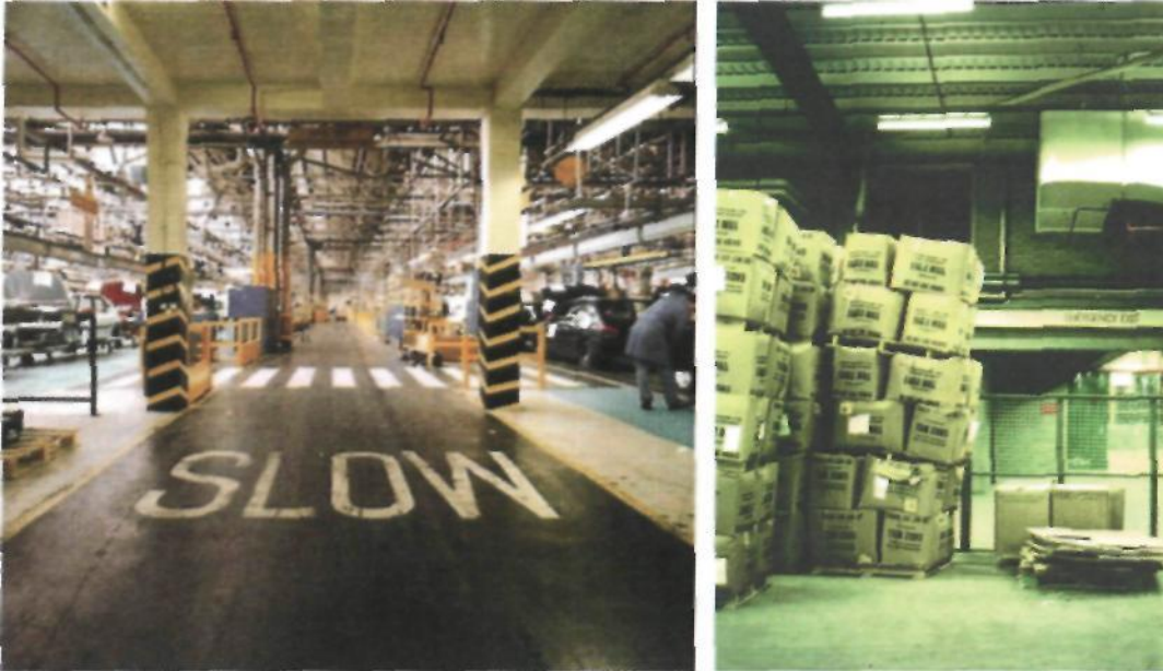
Figure - Internal roadway with appropriate markings (b) Unsafe stacks of heavy boxes.
